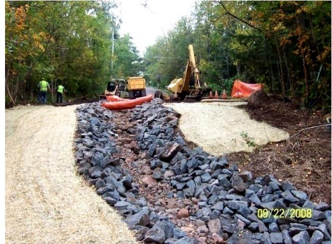
*This rock chute cleans and cools down runoff before it enters Miller Creek at 22<sup>nd</sup> Ave. W.*
