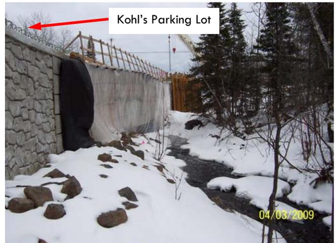
*A new retaining wall was constructed along Miller Creek below the Kohl's parking lot during construction near the Mall.*
