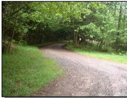
**Building:** On steep slopes, meander your driveway (snake it down the hill in an "S" curve, instead of a straight line). This gives water several places to veer off the driveway, so it won't sheet down in a straight line (taking your gravel with it). Installing water bars, dips,
