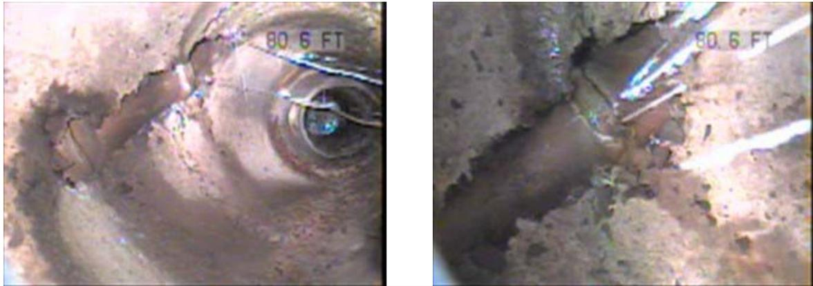
These images are video clips from the sewer cam. On the ceiling of the main stormwater drain tunnel you can see a dark colored pipe that is the much smaller diameter sanitary sewer line. Most of the white streaks are dripping water
